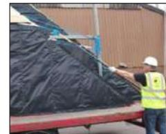
**8. Safety Area** Forked equipment will then lift the panel from the bed of the trailer. Given the weight and shape of panel it is essential that the danger area in front of the panel is kept clear of all personnel. NEVER stand in the danger area where the panel could potentially fall or swing. Do not allow any others to enter the danger area.
