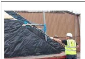
8 The crane will then lift the panel from the bed of the trailer. Given the weight and shape of panel it is essential that the danger area in front of the panel is kept clear of all personnel. NEVER stand in the danger area where the panel could potentially fall or swing. Do not allow any others to enter the danger area.
