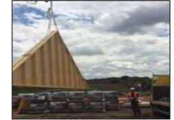
**7. Release Panel.** The Lifting equipment will then take up any further slack of the lift. The driver will cut the individual blue rope attaching the panel to the vehicle centre bars. This must be carried out from a safe position using a telescopic cutting staff
