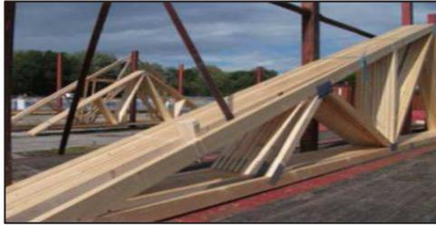
9. The customer team will then take hold of the truss while the driver cuts the blue rope. Once the blue rope has been cut the team will then off load the truss in a safe manner. Proceed with this recommended method for the remaining trusses.
