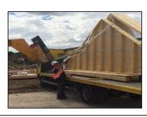
7. Release Panel. The Lifting equipment will then take up any further slack of the lift. The driver will cut the individual blue rope attaching the panel to the vehicle centre bars. This must be carried out from a safe position using a telescopic cutting staff
