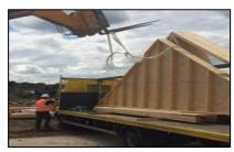
4 Slings Drivers and site staff are not permitted to access lorry bed during unloading. Spandrel Panels will arrive preslung with appropriate lifting slings. It is recommended Forked equipment is fitted with appropriate Crane Hook attachment. Where not available, forks must be
