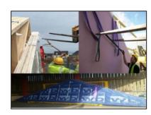
8. Safety Area Forked equipment will then lift the panel from the bed of the trailer. Given the weight and shape of panel it is essential that the danger area in front of the panel is kept clear of all personnel. NEVER stand in the danger area where the panel could potentially fall or swing. Do not allow any others to enter the danger area.
