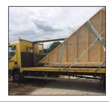
**6.**Lifting. The Lifting equipment will then take up the slack of the lift. On instruction from the site responsible person the driver will release the transport straps on the side being unloaded. Guide ropes may also be attached to pre-installed straps along bottom chord.
